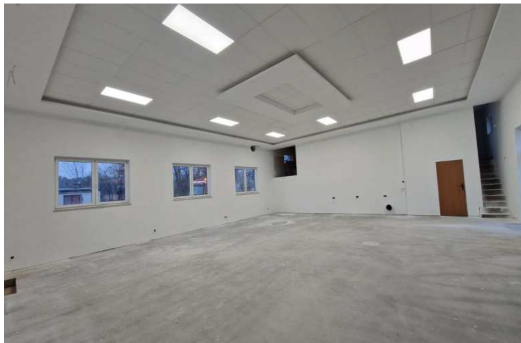
Remont remizy OSP Kawki
